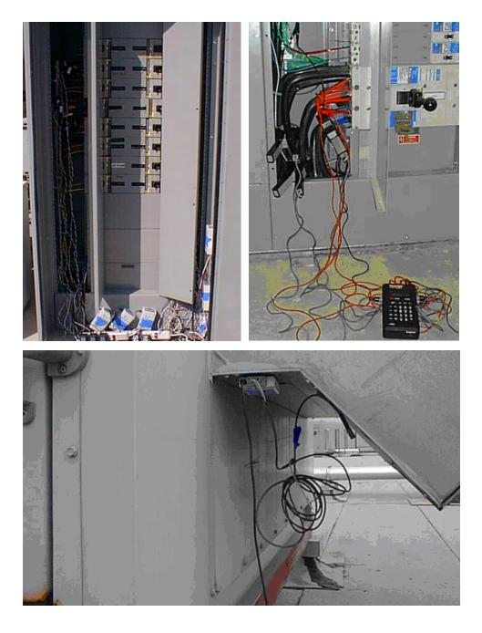
Figure 4: Two kinds of power meters deployed to trend panels (five circuits on right, one on left). Note: safety tape and barriers are not shown.
