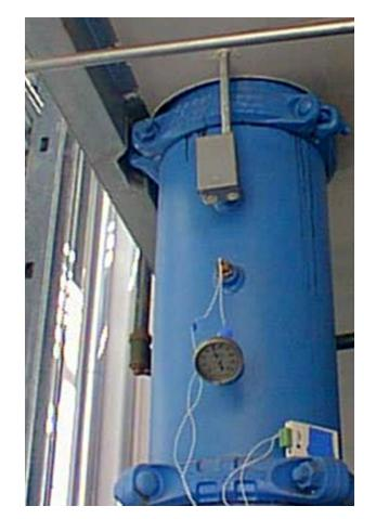
Figure 6: Ultrasonic 'strap-on' temporary flow meters
