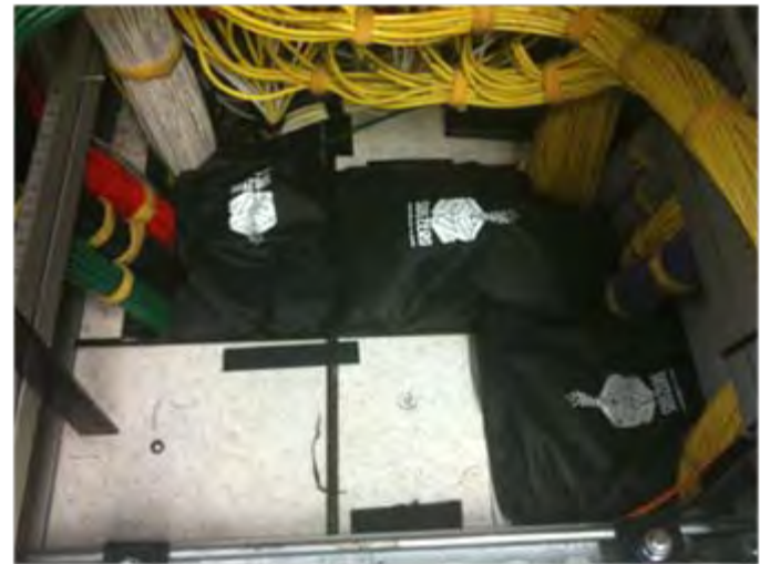
Sealed cable penetration
