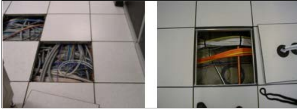
Figure 6.5: Poor (left) and Good (right) Cable Management (ANCIS Incorporated)
