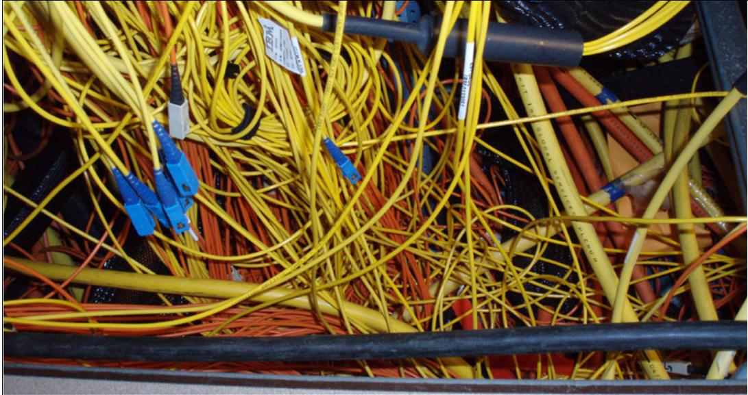
Figure 4-3 Under-floor blockages
