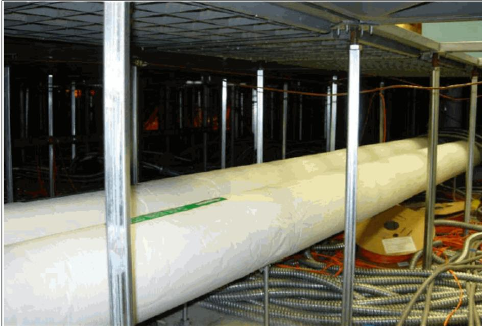
Figure 4-5 Under-floor view with chilled water pipes
