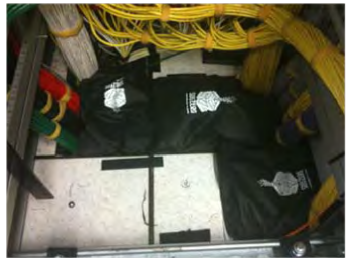
Sealed cable penetration
