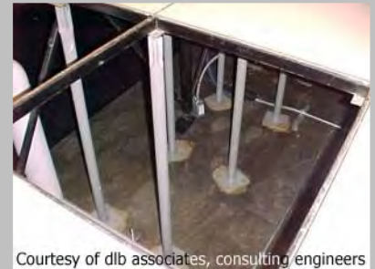
Empty Floor & Ceiling Cavities
