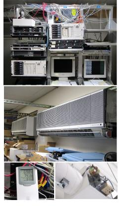
air-side economizer could be installed. This could be in the form of an exhaust fan removing heat in one portion of the room and an opening in another location allowing cool, outside air to enter; or it could be in the form of a fan coil or CRAC/H with air-side economizer capability. Depending on the climate zone in which the server closet is located, this strategy can save a significant amount of energy by reducing compressor cooling energy use.
