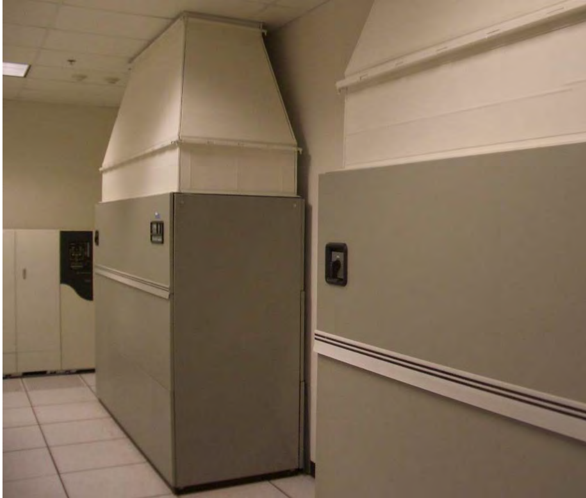
Return air duct on top of CRAC unit connects to the return air plenum.
