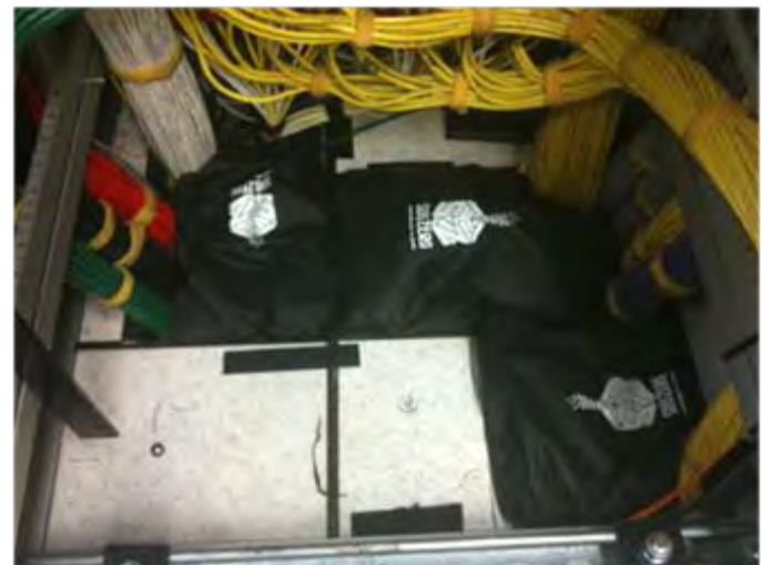
Sealed cable penetration
