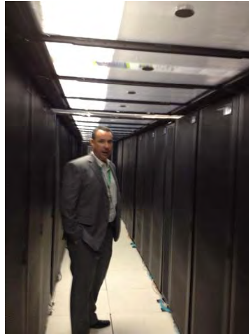
APC Hot Aisle Containment (with in-row cooling)
