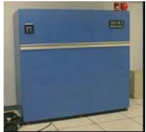
Figure 12 Typical CRAC unit
