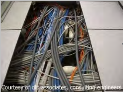
Congested Floor & Ceiling Cavities
