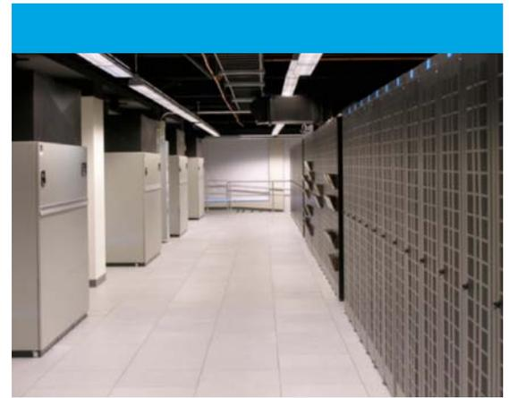
The Sybase data center in Dublin, California, is a physically well-organized and energy-efficient environment. Implemented cooling plant and air management measures at Sybase allowed raising the chilled water temperature from 43°F to 52°F, which saved at least 15% of the chiller energy. The room temperature was also raised from 69°F to 74°F.
