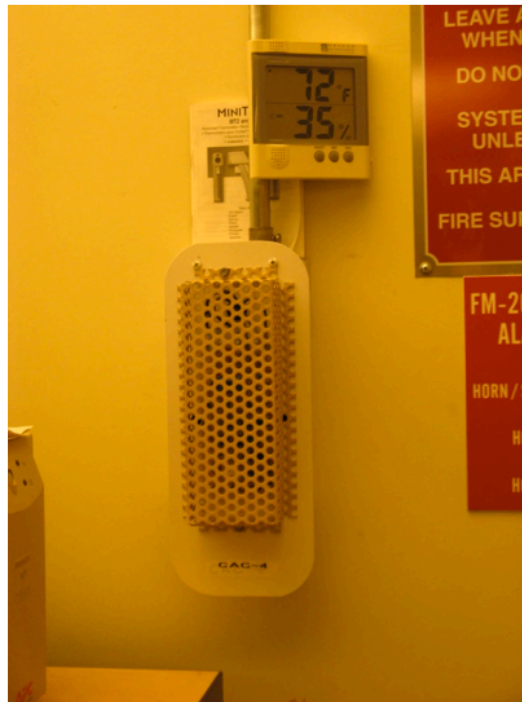
Figure 7: City of Walnut Creek -- Temperature and Relative Humidity Sensor Sets
