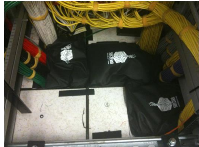
密封的电线穿墙 Sealed cable penetration
