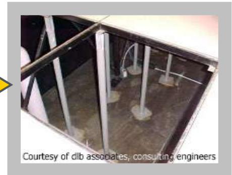
Empty Floor & Ceiling Cavities
