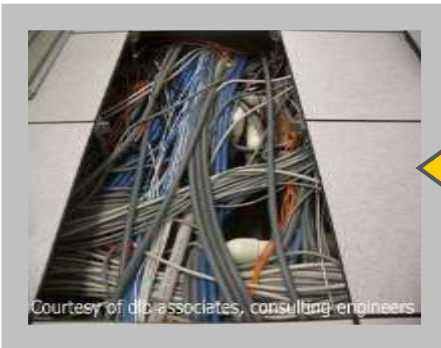
Congested Floor & Ceiling Cavities
