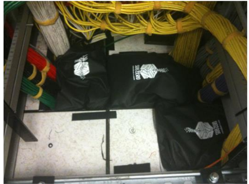
Sealed cable penetration
