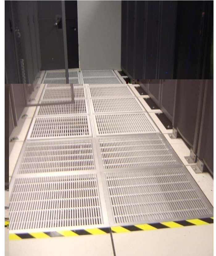
High-flow tiles reduced air pressure
