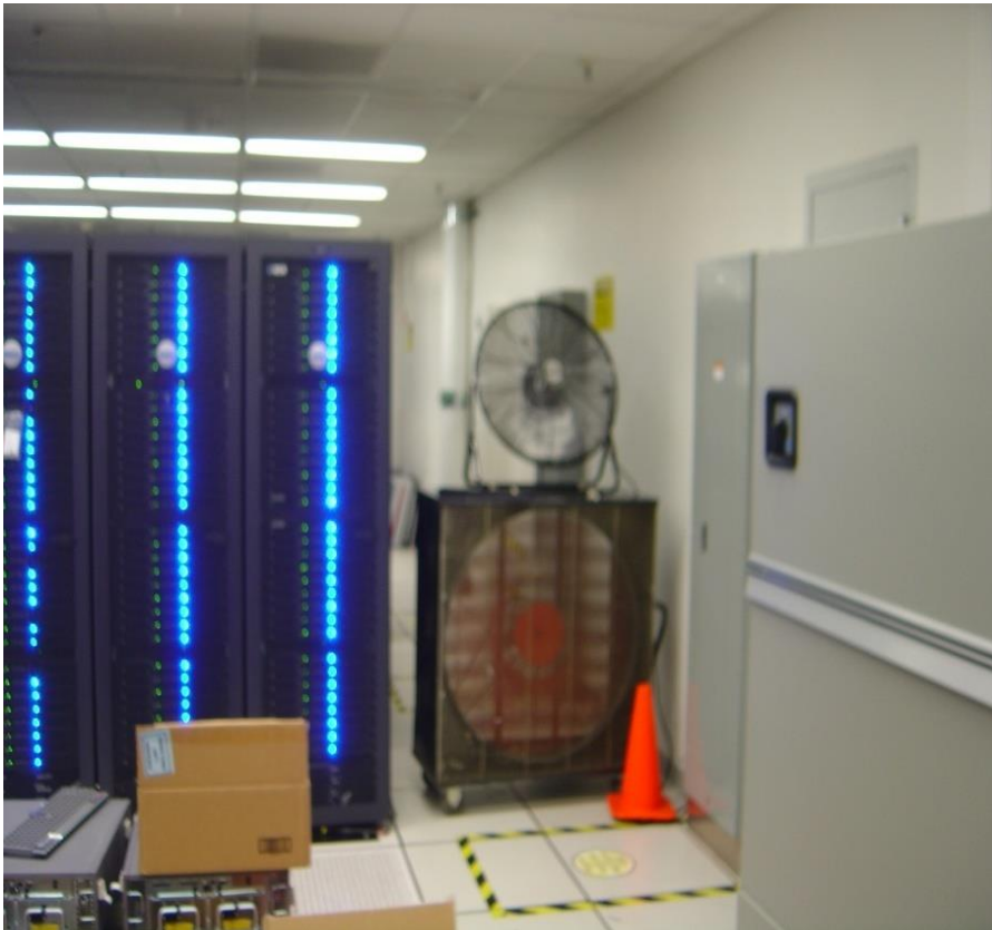
Fans were used to redirect air
