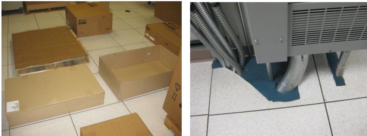
Figure 32: Covered Perforated Tiles and Conduit Penetration
