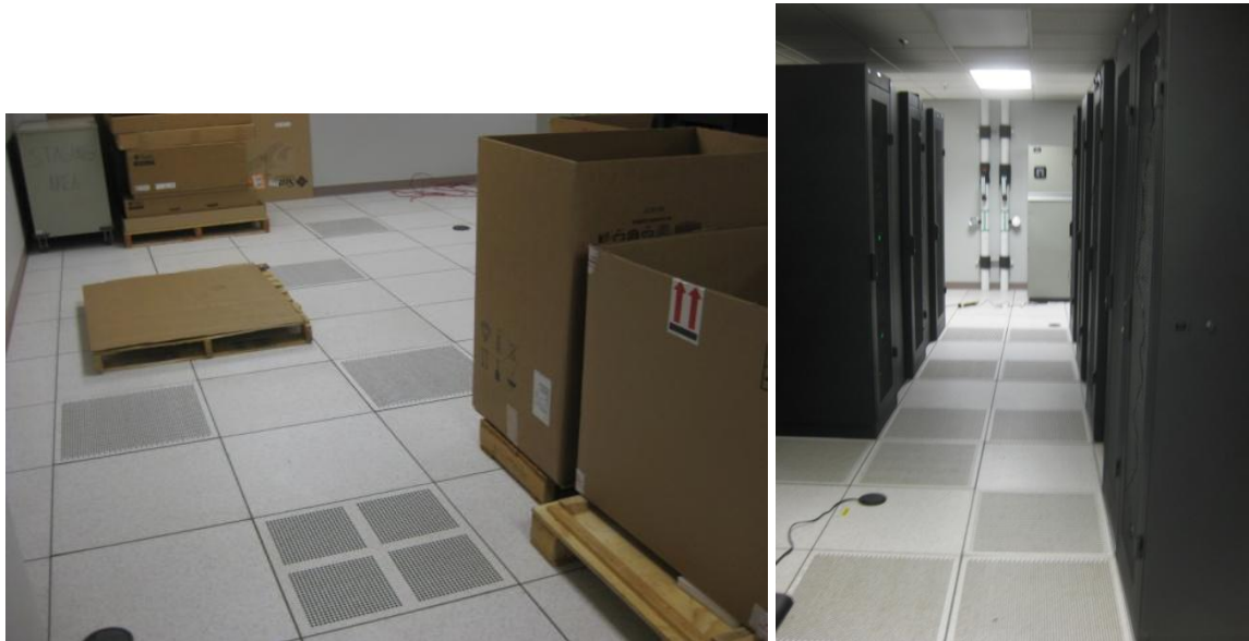
Figure 14: Examples of Misplaced Perforated Tiles
