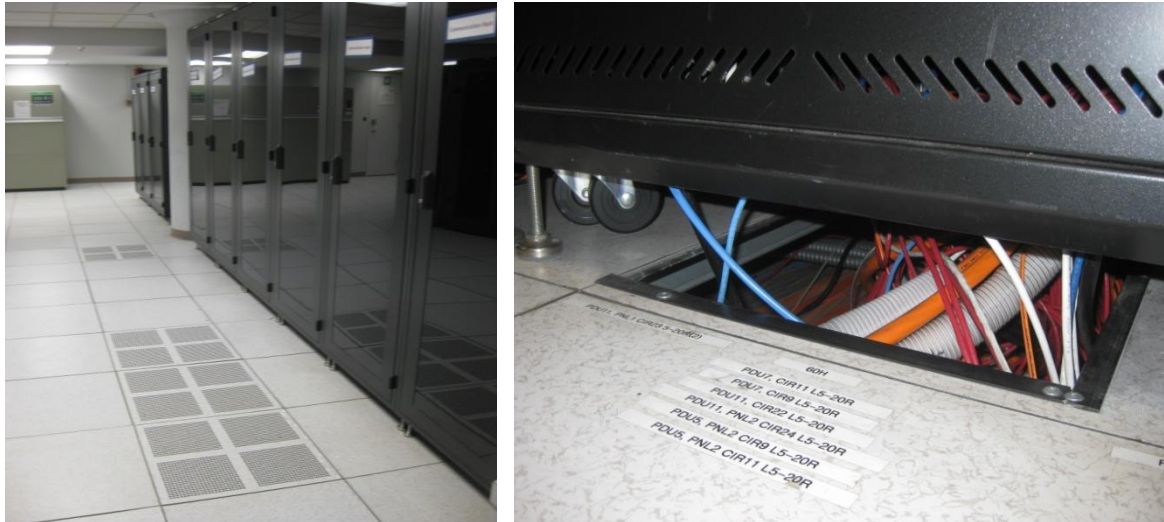
Figure 16: Perforated Tiles in Front of Cabinets and Openings for Cables
