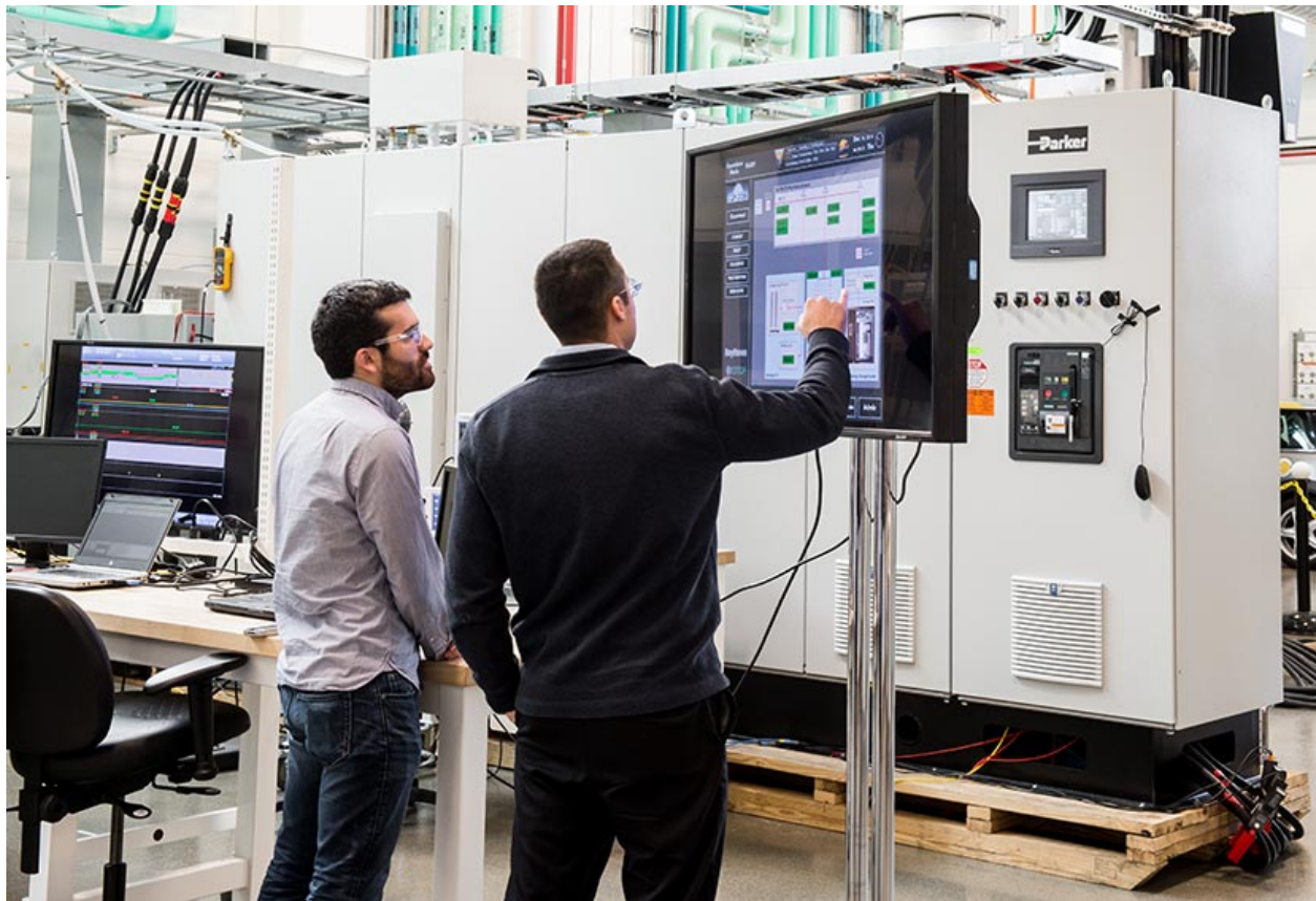
NREL and Raytheon performed system-level testing for MCAS Miramar on a simulated microgrid at NREL's Energy Systems Integration Facility in 2014. Photo by Dennis Schroeder, NREL
