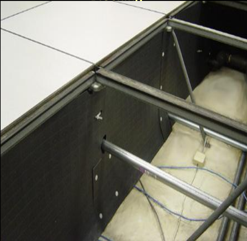
Unused Area Under raised floor Blocking
