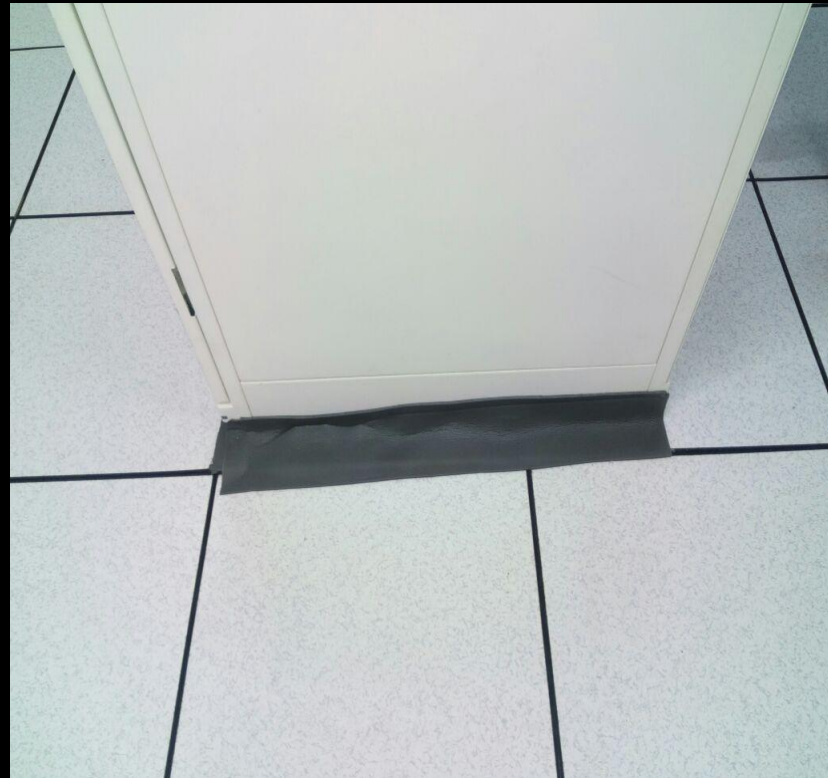
PDU side gap Blocking
