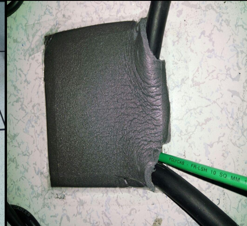
Cable Entry cut outs Blocking
