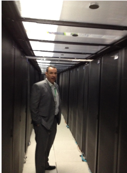
APC Hot Aisle Containment (with in-row cooling)
