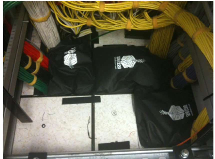
Sealed cable penetration
