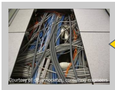
Congested Floor & Ceiling Cavities
