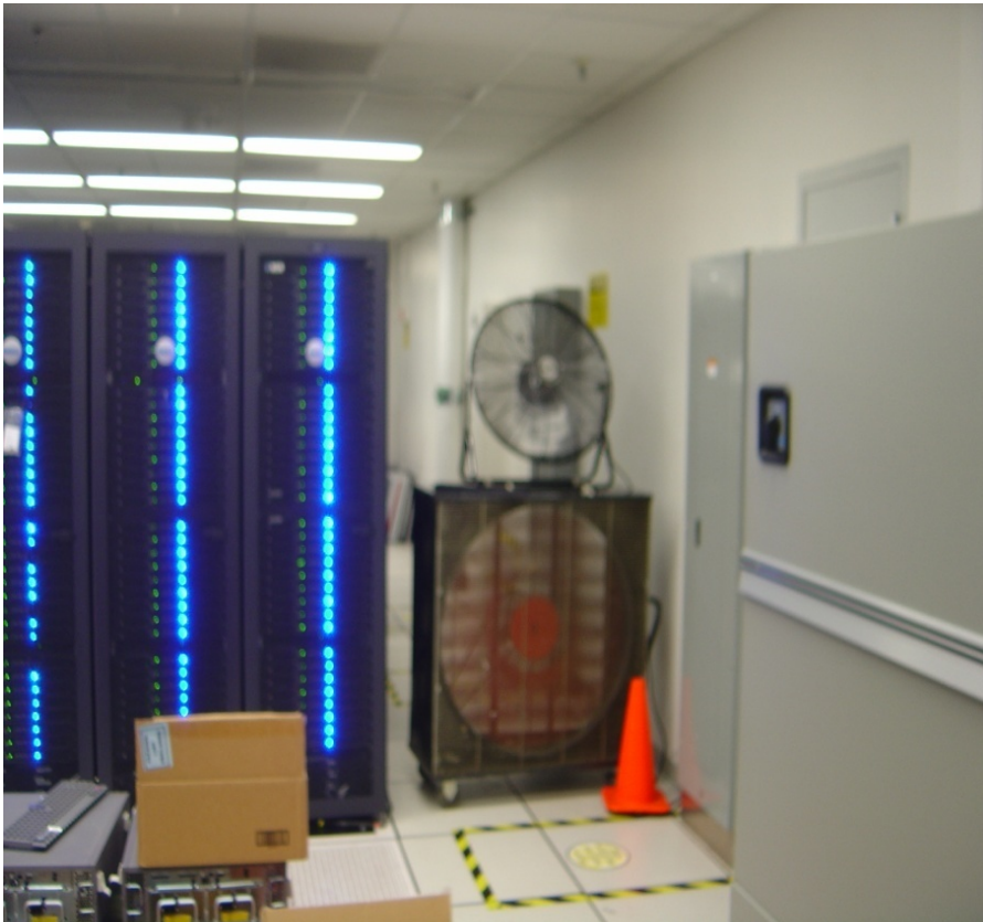
Fans were used to redirect air
