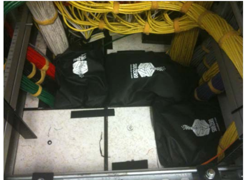
Sealed cable penetration
