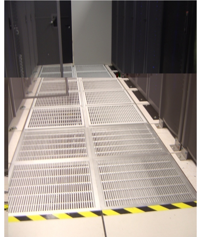
High-flow tiles reduced air pressure
