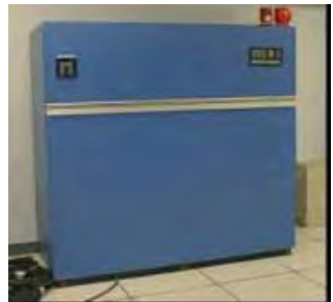
Figure 12 Typical CRAC unit
