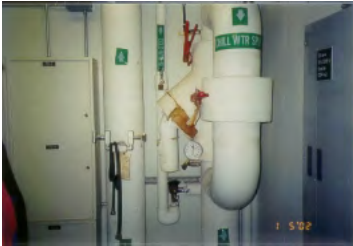
Figure 9 Chilled Water Piping
