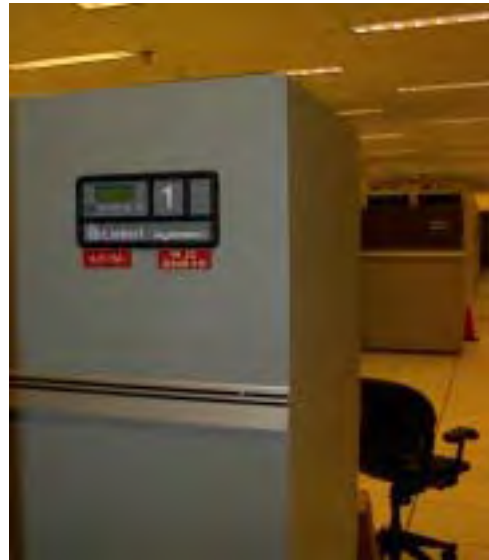
Figure 1 CRAC Unit
