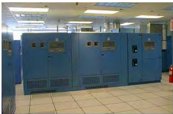
Figure 10 An older UPS system
