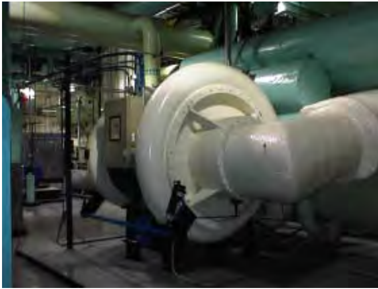
Figure 13 Centrifugal Chiller
