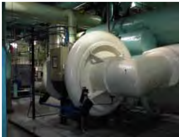
Figure 2 Centrifugal Chiller
