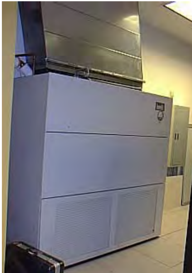
Figure – Data Center Air Handling Unit
