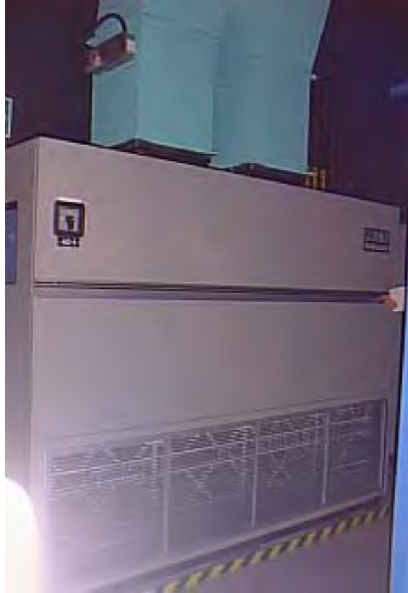
FIGURE 2. DATA CENTER CRAC UNIT
