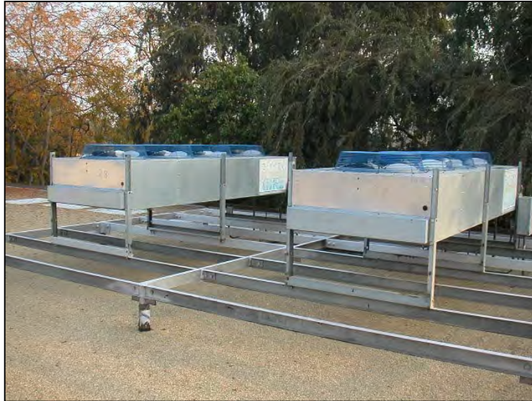
Figure 12. Air-Cooled Condensers on Roof
