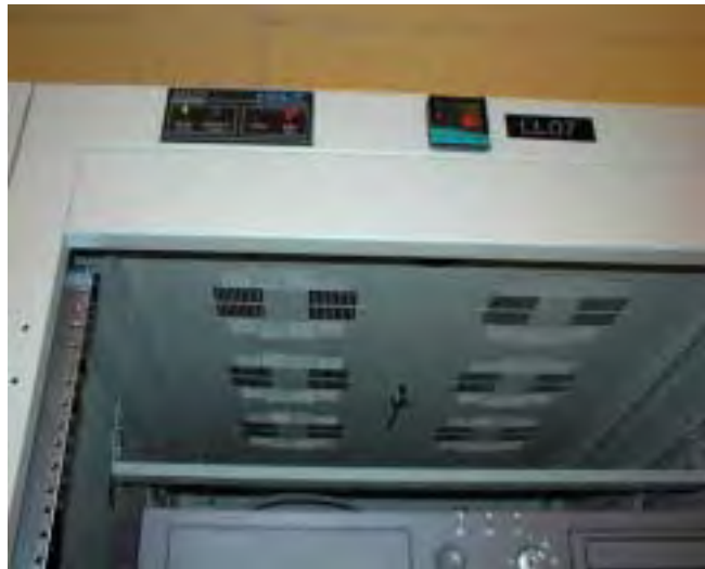
Figure 7 Top of cabinet showing fans
