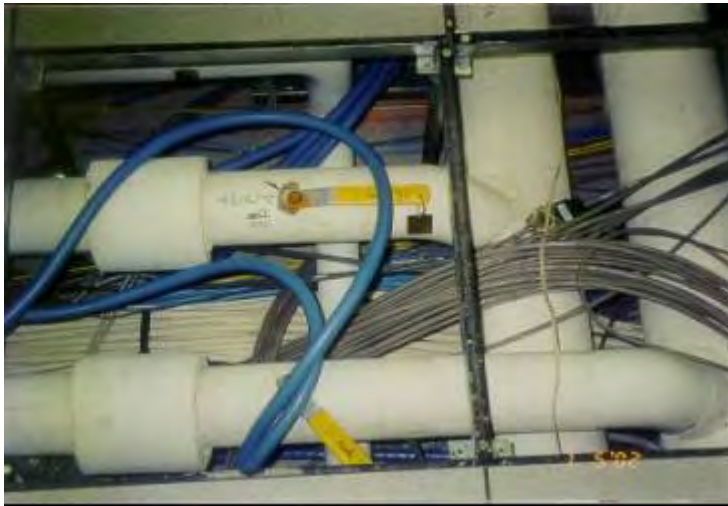
Figure 14 This under floor area in the NY Data Center severely restricts air flow
