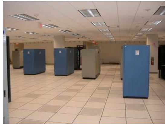
Figure 4: Open floor tiles.
