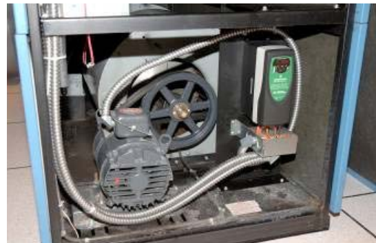
Figure 5: VFD installed.
