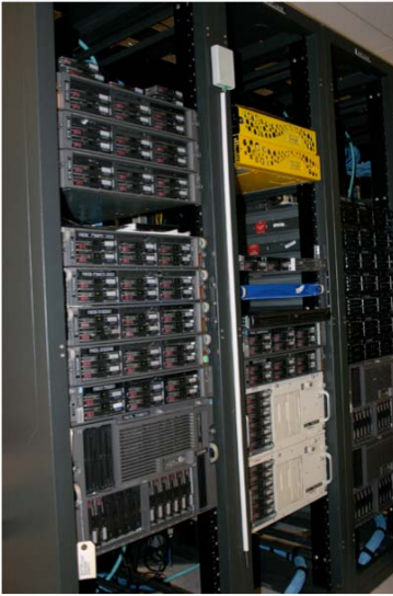
Figure 2: Inlet air sensor.
