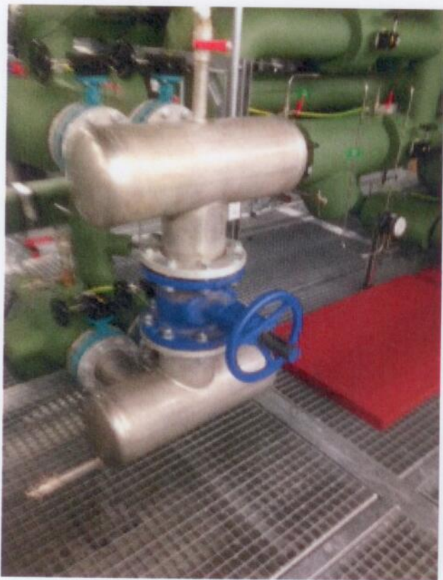
Figure 6. Photograph showing the pipework, prior to lagging, for one of the primary- to secondary-side heat exchanger by-passes, including cross-connect valve.
