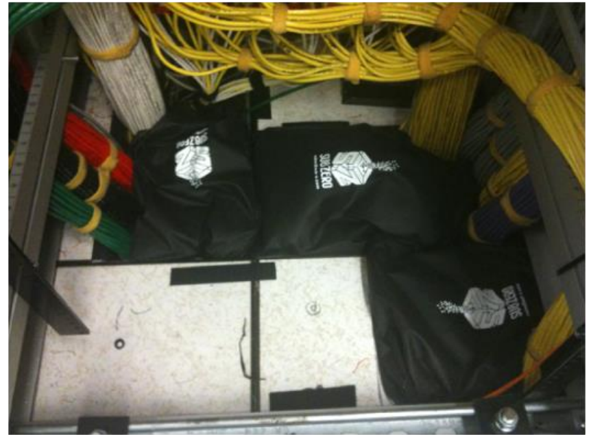
Sealed cable penetration
