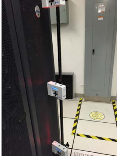
Figure 19: PurkayLabs: Leaning rod due to uneven floor.
