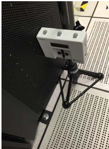
Figure 18. PurkayLabs: No obstruction. Units can be placed close to the rack fronts.
